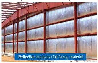
While reflective insulation materials can be used in any climate, it is most effective in southern states where excessive heat can send energy cost soaring. Reflective insulation materials are tested under the ASTM 1224 Standard Specifications for reflective insulation for building applications. Included in these criteria is a fire test. ASTM E84-09 and ASTM E2599 require reflective insulation to have a flame spread rating of 25 or less, and a smoke development rating of 50 or less.
