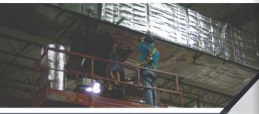
rFOIL® BIG-8 is specially designed to reduce radiant heat gain/loss in all residential and commercial duct applications. rFOIL® also helps control condensation by providing an airtight thermal break around duct work.
