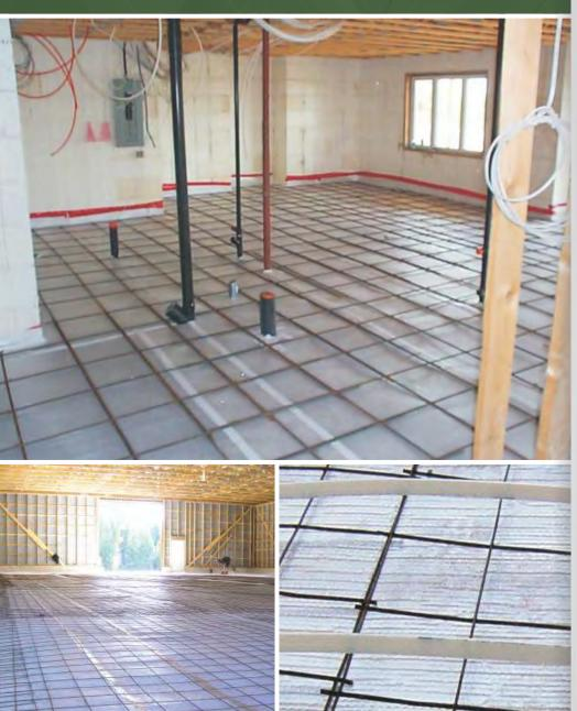
**rFOIL** Standard Concrete Underpad is an outstanding reflective insulation and puncture-resistant vapor barrier. It is composed of a double layer of high-strength polyethylene bubbles sandwiched between a layer of highly reflective metalized film and a clear polyethylene sheet.
