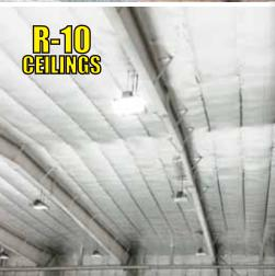
**rFOIL**® reflective Insulation is a layer of polyethylene bubbles bonded to and sandwiched between a radiant barrier metalized film surface and a white polyethylene sheet.
