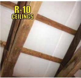
**rFOIL**® reflective Insulation is a layer of polyethylene bubbles bonded to and sandwiched between a radiant barrier metalized film surface and a white polyethylene sheet.
