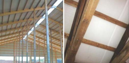
**rFOIL**® reflective Insulation is a layer of polyethylene bubbles bonded to and sandwiched between a radiant barrier metalized film surface and a white polyethylene sheet.
