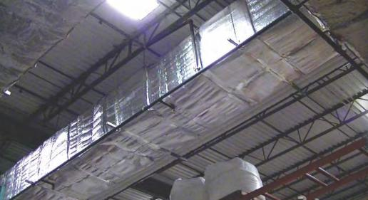
**rFOIL®** Reflective Duct Insulation is a double-layer of polyethylene bubble, bonded to and sandwiched between two highly reflective metalized film surfaces.
