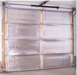
**rFOIL**® reflective Insulation is a single or double layer of polyethylene bubbles bonded to and sandwiched between two highly reflective metalized film surfaces.
