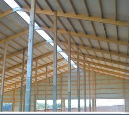
**rFOIL**® reflective Insulation is a layer of polyethylene bubbles bonded to and sandwiched between two radiant barrier metalized film surface sheets.
