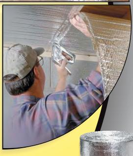
**rFOIL**<sup>™</sup> reflective Insulation is a single or double layer of polyethylene bubbles bonded to and sandwiched between two radiant barrier metalized sheet.
